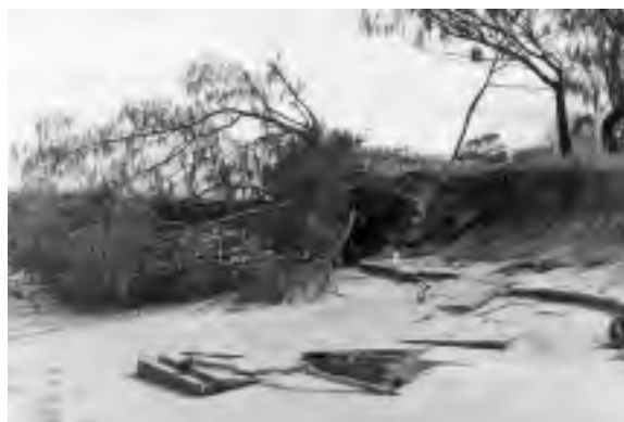
Figure 2.5 Example of recent bank recession of the north bank of Middle Creek, showing concrete stairs once used to access the beach from the top of the erosion bank some 15m away from the contemporary section. Facing northwest.
