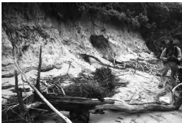
Figure 12.3 General view of steep c.2m high erosion bank at the southern end of Eurimbula Site 1 fronting Round Hill Creek. Facing northwest.
